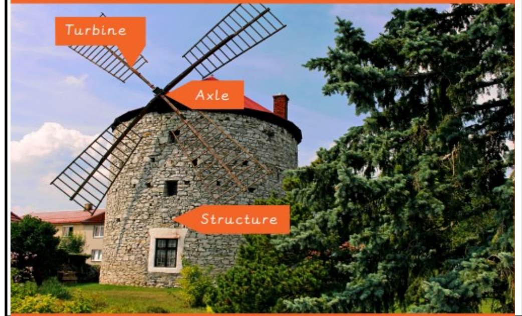
The three main parts of a windmill:
